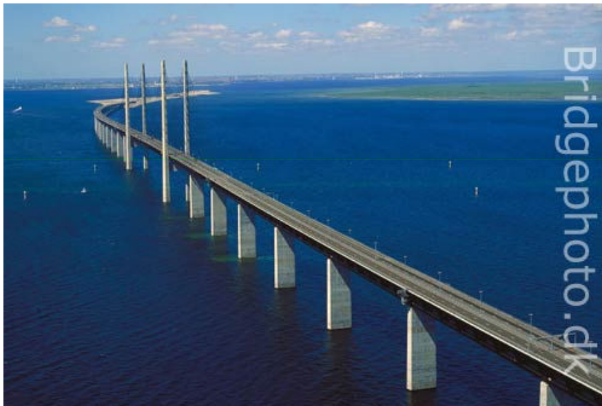
The Øresund Bridge
